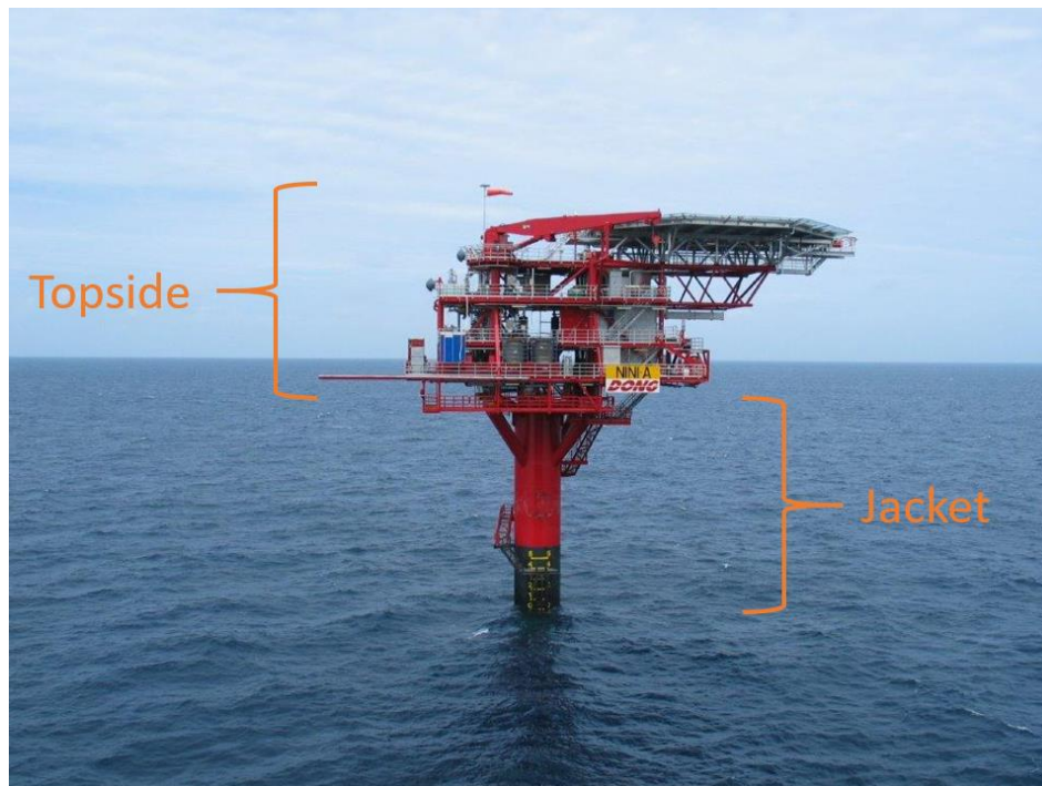
Figure 4-4 Topside and jacket extend to the seabed of the Nini A platform (water depth approx 60 m).
