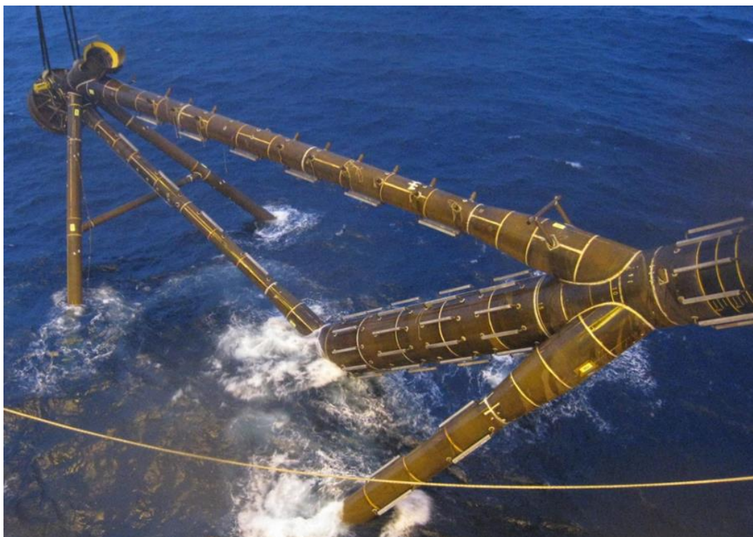
Figure 18-3 Jacket structure during installation.
